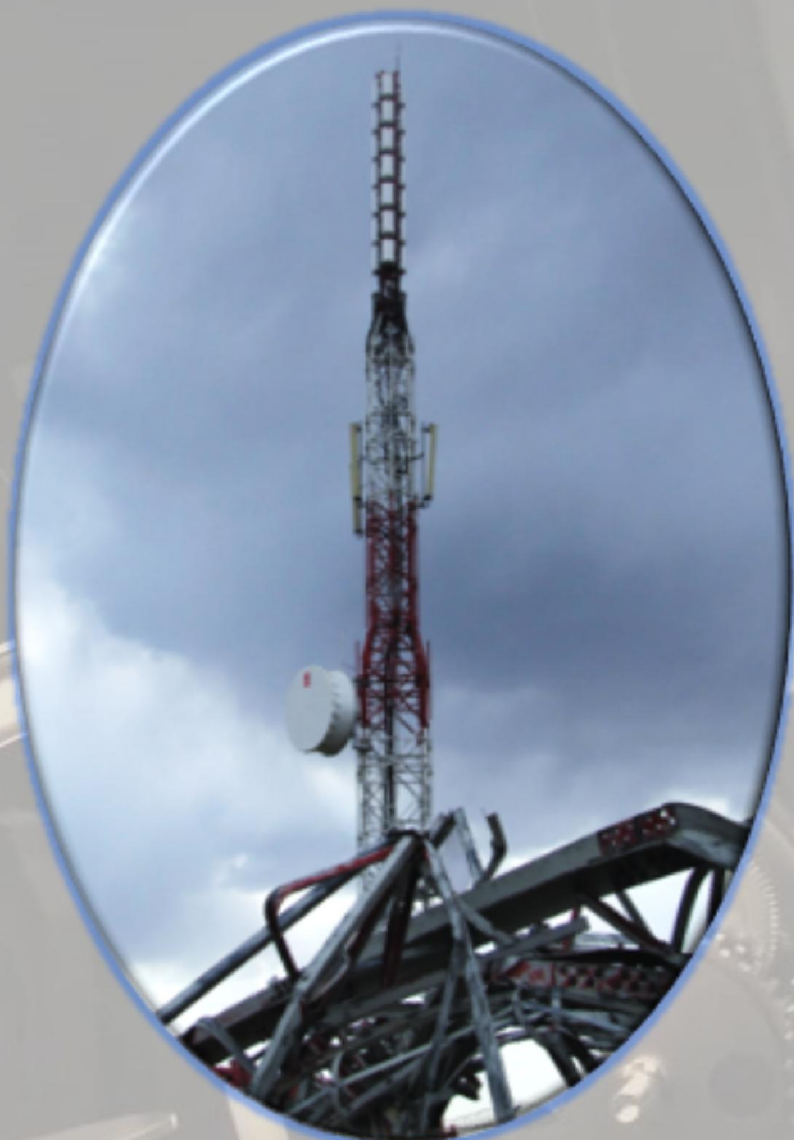
Broadcasting Towers (Redesign & Repair)
