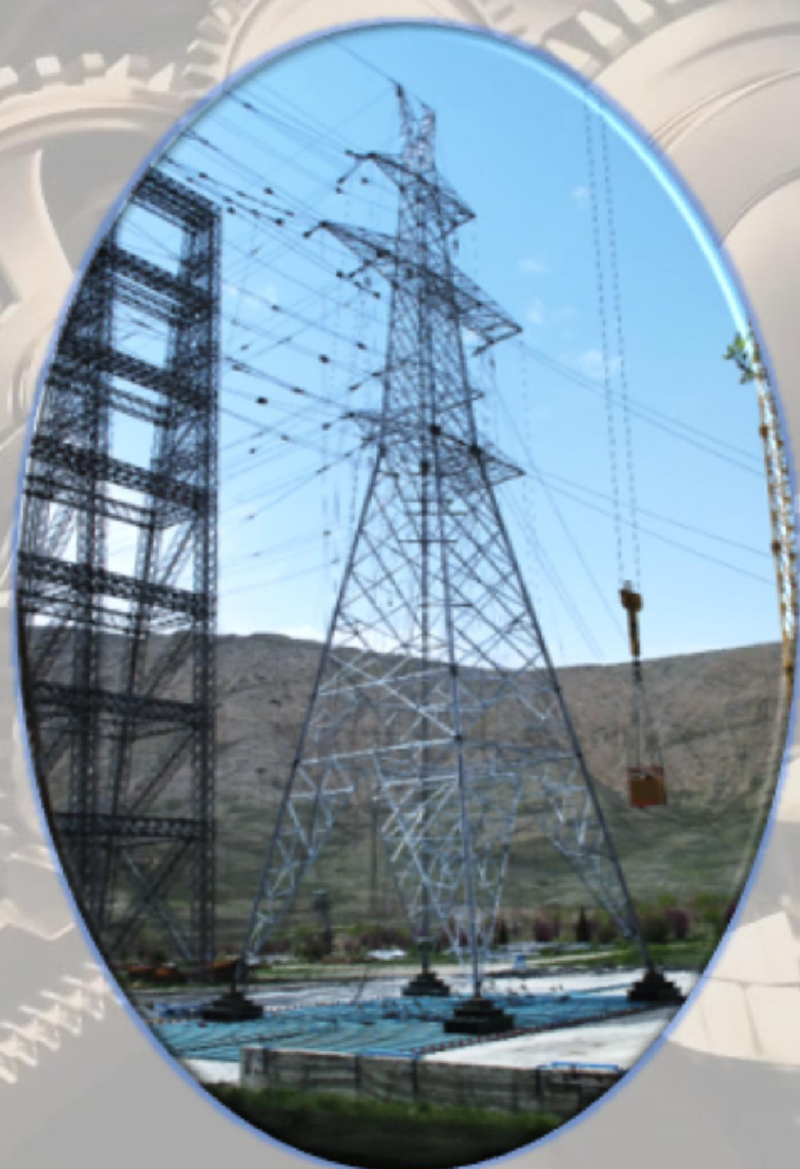
Transmission Towers (Optimization & Upgrade)
